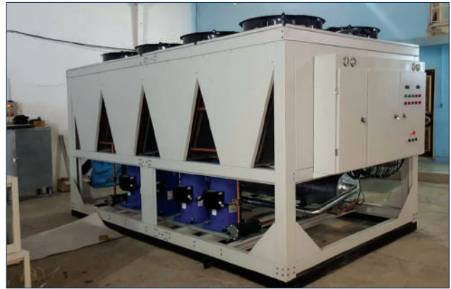
Figure 39. Example of air-cooled chiller.
