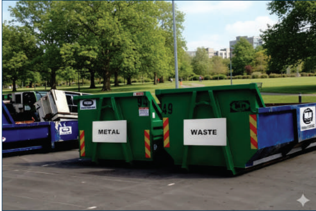
Figure 64. Segregation of construction waste.
