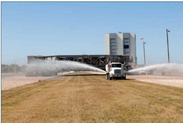
Figure 62. Watering the ground to prevent dust rising from the soil.
