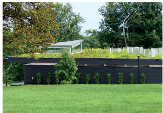
Figure 28. Example of an extensive green roof: Jesuit Center Garden Roof at Fairfield University in Fairfield, Connecticut, USA.
