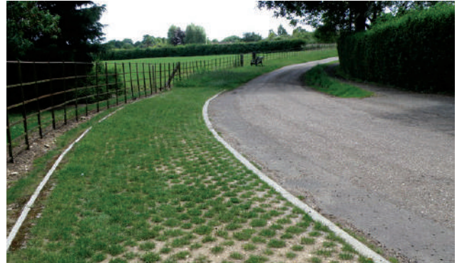
Figure 11. Example of pervious paving.
