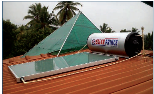
Figure 46. A typical solar hot water system – collector plate with the cylindrical hot water tank.
