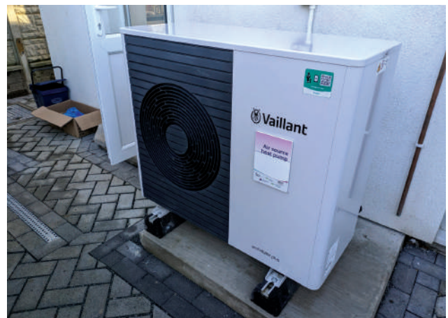
Figure 47. Image of a typical air source heat pump.
